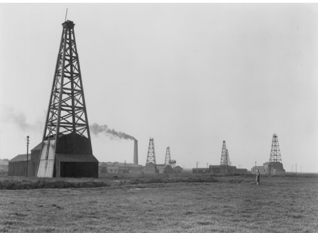
Drilling Rig near Greatham (IH)
