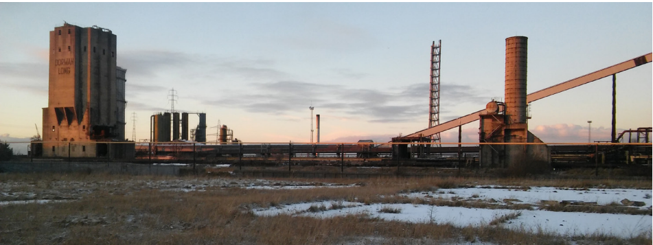
Coal bunker on the left and part of coke works on the right (AJB)
