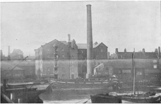
1840 Flour Mill on Stockton Riverside c1905
