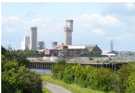
View from riverside of two silos with the tall prilling tower behind
