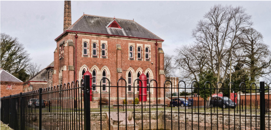
Tees Cottage Pumping Station
